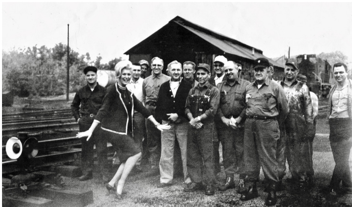
Osceola Railyard workers take a break to pose with Miss Pennsylvania Railroad in front of the enginehouse during the last years of the railyard.
