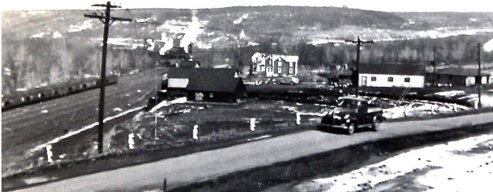
Looking over the Moshannon Coal Company mining offices near Klondike toward the Osceola Yard enginehouse and roundhouse.
