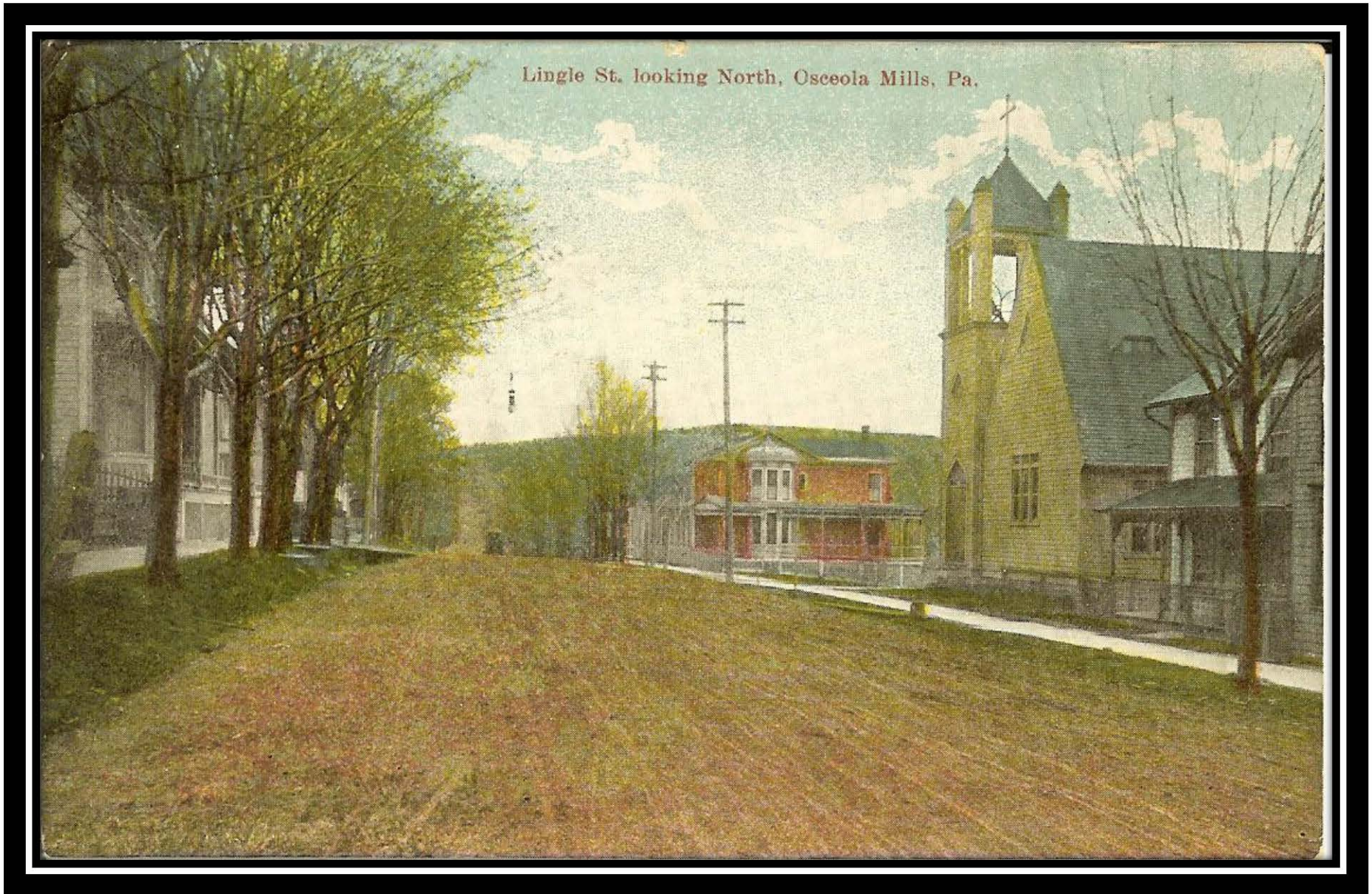
Figure 20 -Lingle Street Looking North
