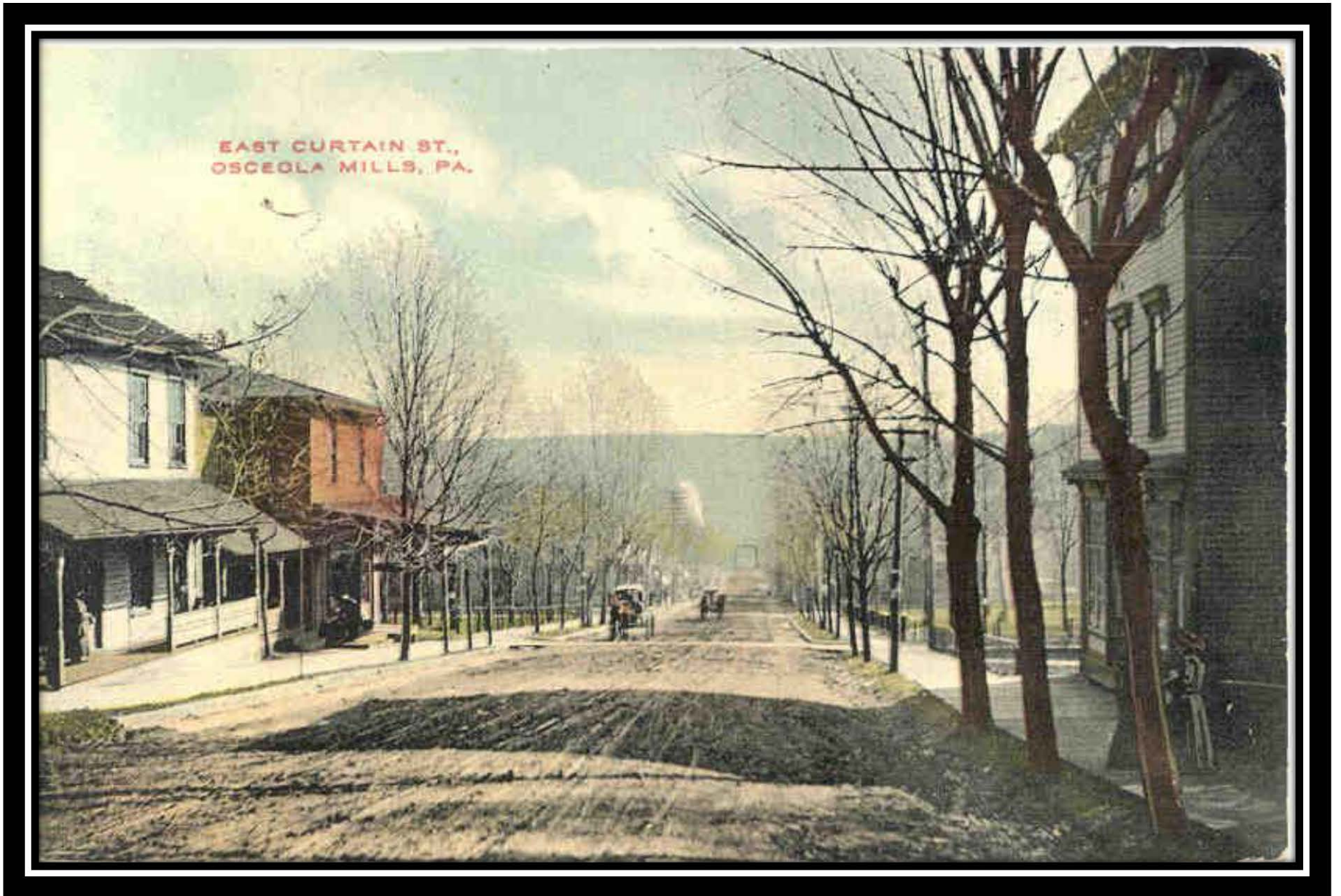
Figure 13 - East Curtin Street
